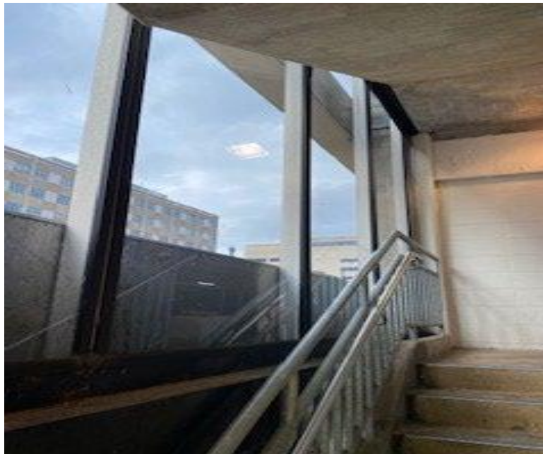
Photograph 6 – A view of the stairwell windows.
